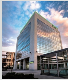
HQ Mansion of DKV, Spain
